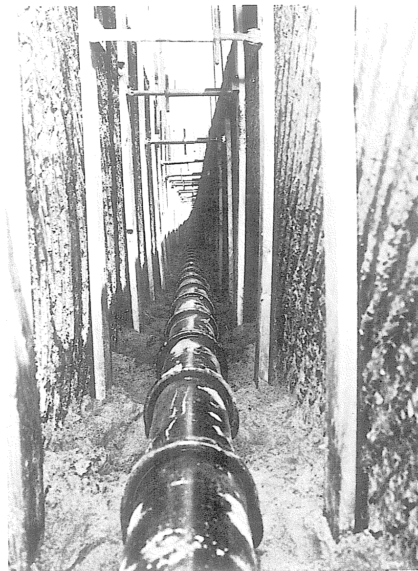
FIGURE 66.—Vitrified clay pipe installation in lightly braced trench.
