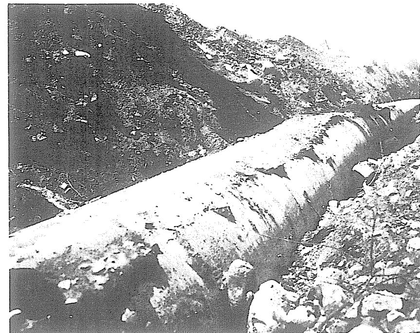
FIGURE 75.—Sewer floated before backfilling was completed.
